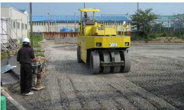
Photo 1. Compaction status of gravel layer
