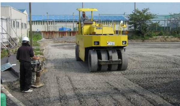
Photo 1. Compaction status of gravel layer
